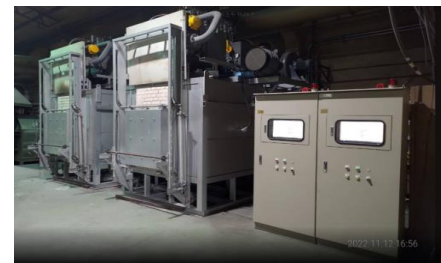
建置蓄熱式燒結爐
